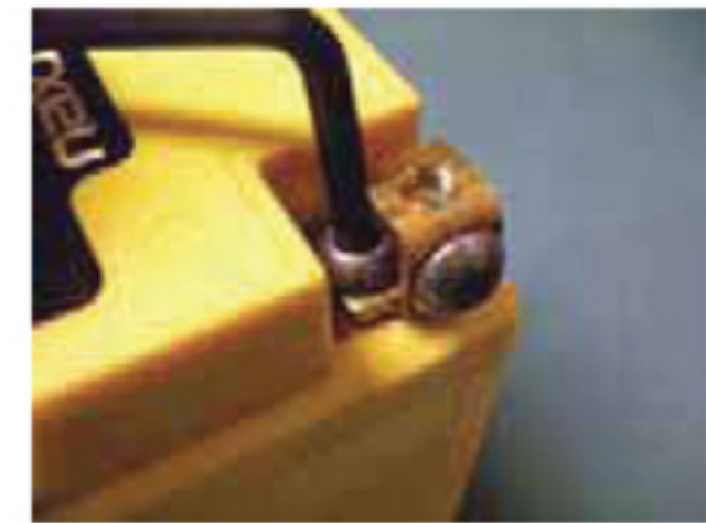
Attaching the terminals
