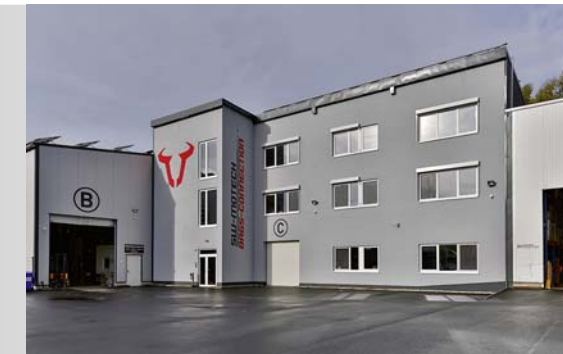
Receiving area/office building, Rauschenberg, Germany
